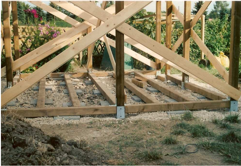
Figure 1.6: Summer house construction
